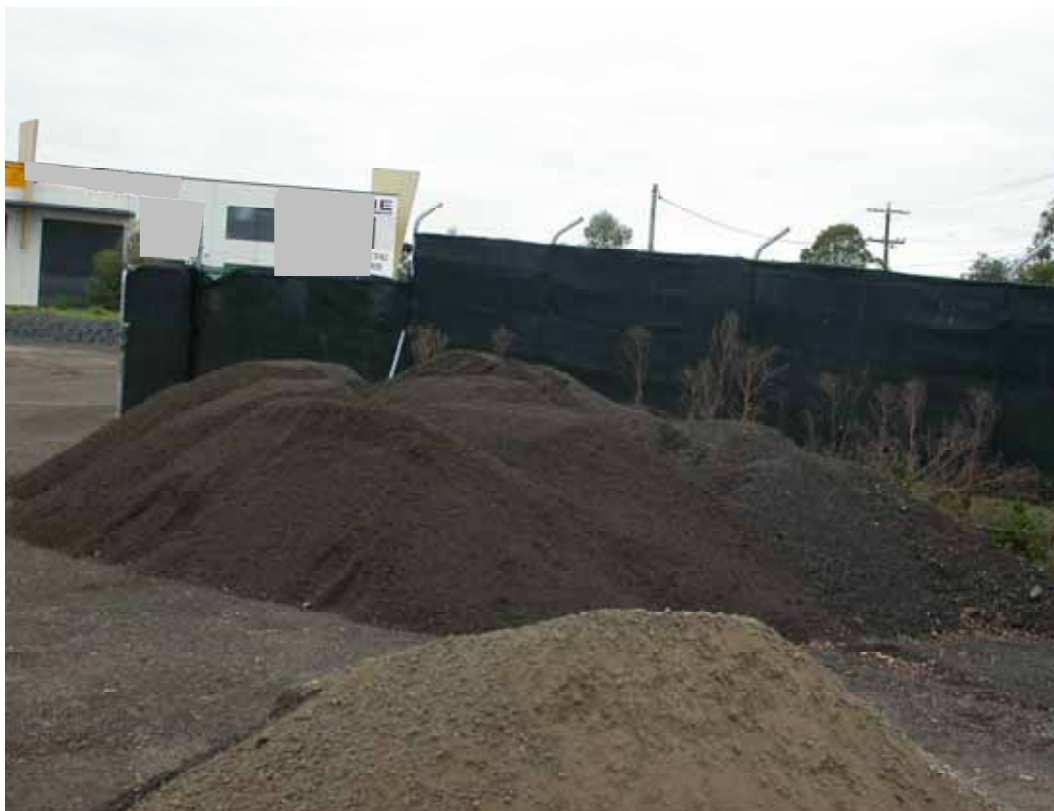
Figure 6. Stockpile infested with weeds
